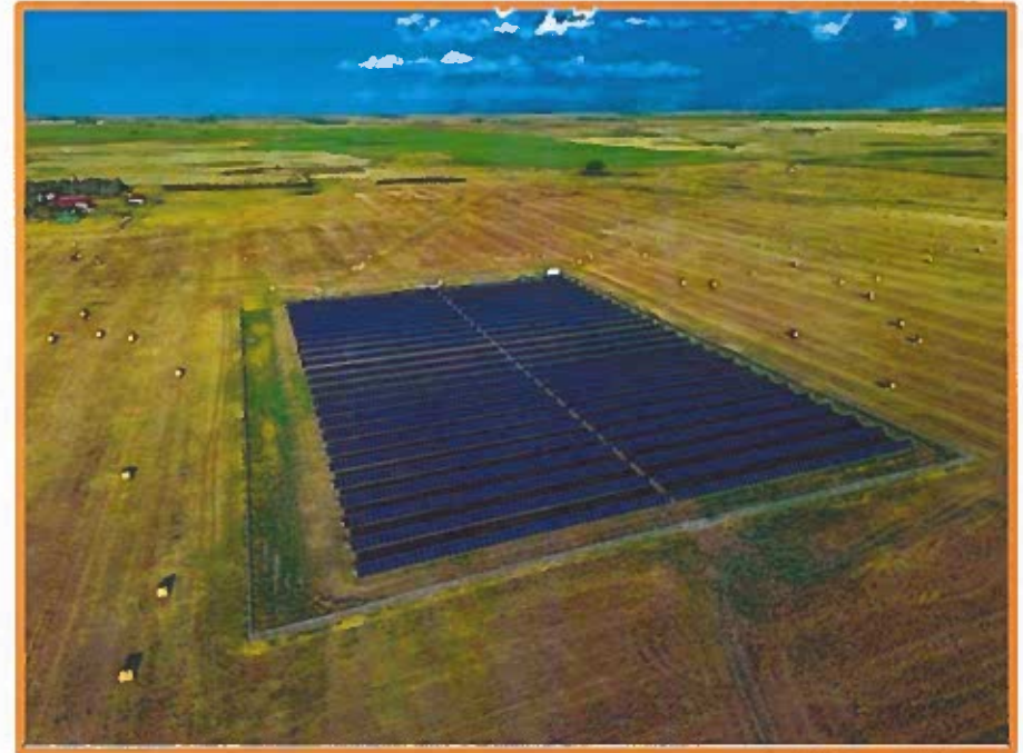
Example of a solar project – Compass Greenfield Development's NM Solar 2020 Inc., Lomond Saskatchewan – approximately 7 acres
