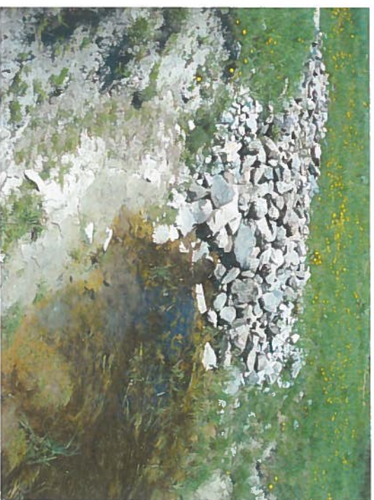
Tile Outlet to Open Channel
