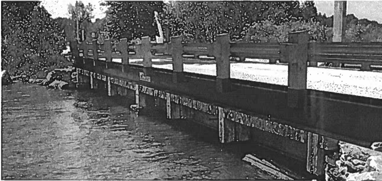
Photo Above - Lessard Modular Bridge Elevation ( Soffit = Existing Bridge Deck). The New bridge would span from bank to bank and wouldn't require the support form the intermediate crib that is mid span in the waterway.
