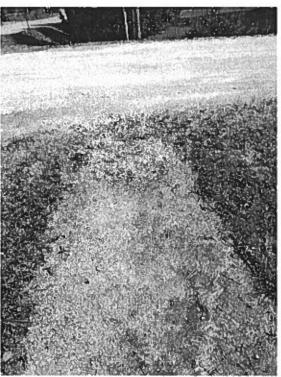
Pea gravel coming of Albert Street on to the sidewalk is a walking hazard as the gravel rolls under foot when one steps down off Albert onto the sidewalk. Mud collects from rains throughout the year as it is washed from the road and surrounding grassed areas along the sidewalk which are higher than the sidewalk itself.
