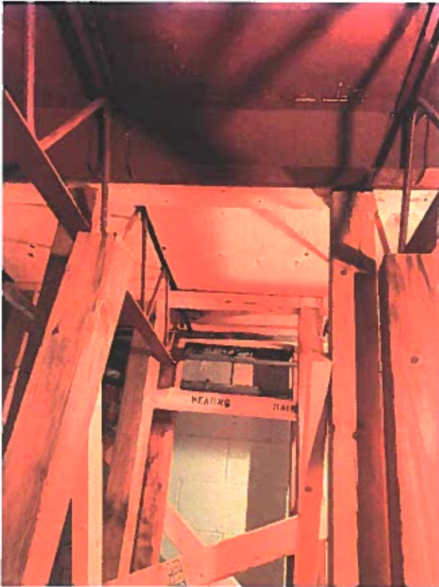
Photograph 7 Basement Wood Shoring under Entrance Vestibule
