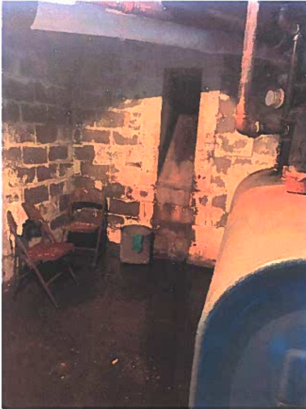
Photograph 1 Basement Water Penetration
