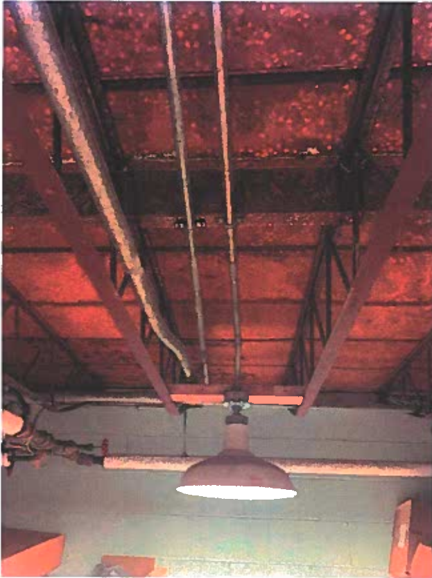
Photograph 9 Rusted Ground Floor Framing
